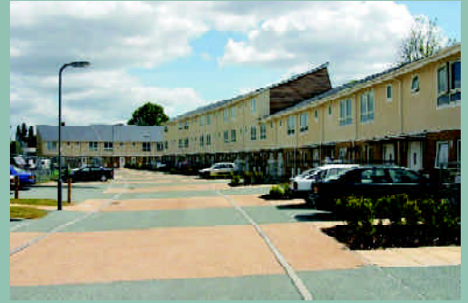
A shared surface for vehicles and pedestrians reduces traffic speeds - Mason Moor, Southampton
