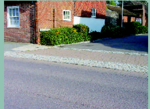
A footpath is demarcated in pavers and setts across an access to a backland development - Petersfield
