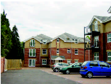
Large areas of hard surfaces without soft landscape give a bleak outlook
