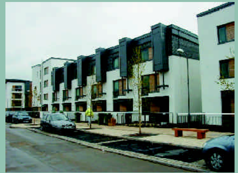
The front boundary walls of this development also provide natural ventilation to the underground car park - Chapel, Southampton
