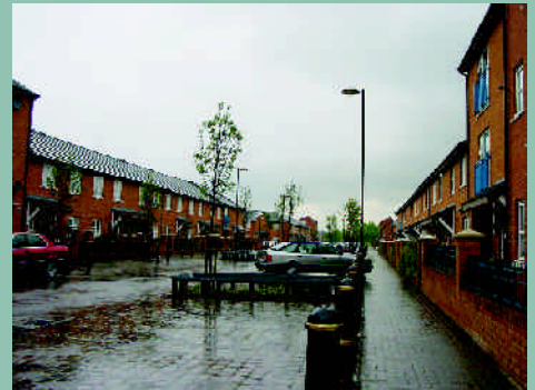
A shared surface with no kerbs and attractive landscape design provides a distinctive character to this street - Birmingham
