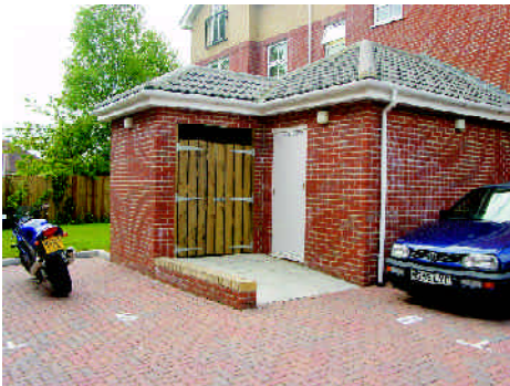
Level access is provided to this cycle store
