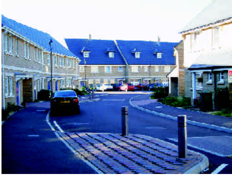
Horizontal deflection features calm the traffic and provide space for on street parking - Northlands Road, Southampton
